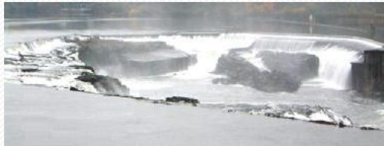
Willamette Falls and Sullivan Hydroelectric Facility.
