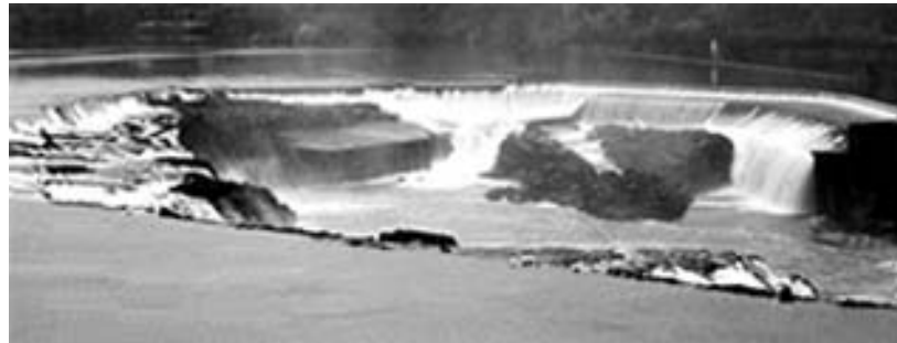
Willamette Falls; Sullivan Hydroelectric Facility.
